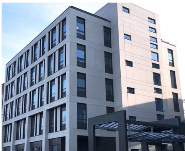
Figure 1. The Cambridge Clinical Research Centre (CCRC), adjacent to Addenbrooke's Hospital, will house the new Neurological Advanced Therapies Treatment Centre comprised of an intraoperative 3T MRI scanner, MRI control room, induction room, recovery room and operating theatre.
